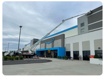
The warehouse's design, with its central main building surrounded by varying lower structures, made reaching the upper facades particularly difficult, especially over the 70- to 80-foot-tall first-floor structures. The on-site JLG lift couldn't achieve 115-foot side reach, prompting the client to seek our expertise.
