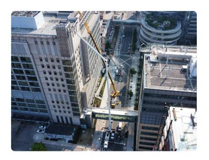
Without a BMU, the only option was to use a crane basket and crane to remove and replace the sign. The old sign was weathered and fragile, requiring gentle care, which made using a crane basket extremely risky.
